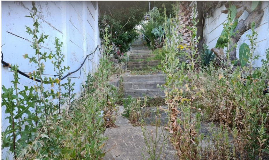
Mossat Lane - before & after
